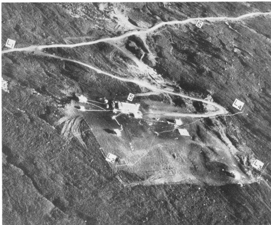
Fig. 2. Aerial view of the observatory, looking north (downslope). L_1 to L_4 are air intake towers. (5) is the main observatory building which houses the analyzer. Aluminum tubing between the towers and the observatory is partially visible. (6) is the road to Hilo. Photograph was taken in August 1962.
